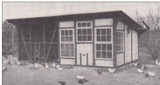
Fig 13: Chick-rearing facility with an enclosed section for colder weather, an open section for warmer days, and an outdoor range (Nussbag, 1957) [28]
