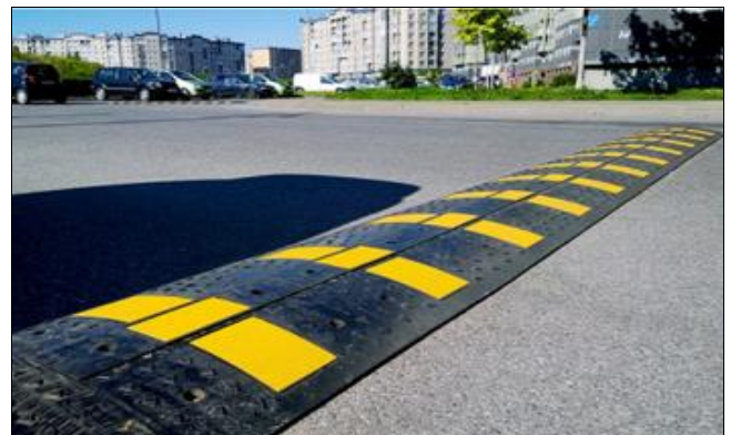
Fig 18: Artificial bumps of the roadway
