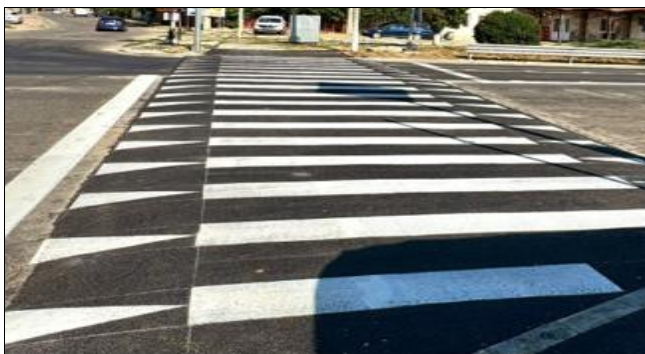
Fig 9: Zebra-type pedestrian crossing, elevated
