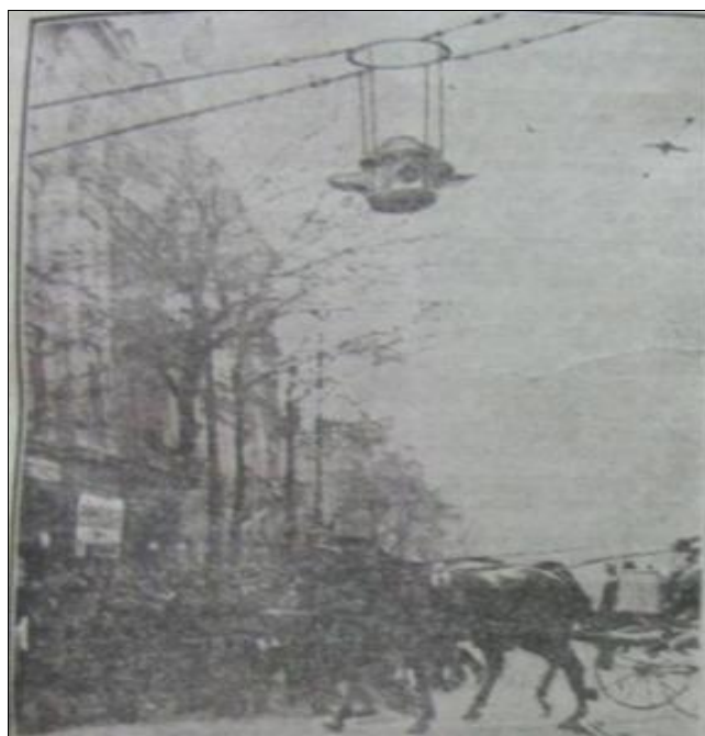
Fig 4: The first traffic light in Bucharest, Romania [5]
