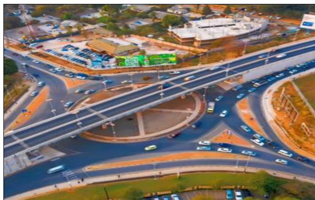
Fig 60: Aerial view of Munali flyover bridge
