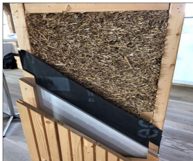
Fig 4: Cut-through of the EcoCocon prefabricated wall exposing various exterior and interior layer's
