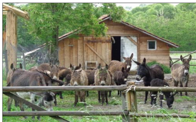
Picture 11: Simple, wooden building (RO) (Foto: M.Urošević)
