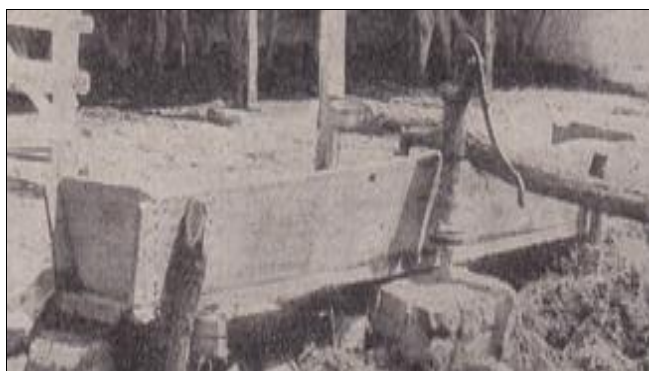
Picture 11: Improperly placed watering trough, right next to the pump (Šterk, 1963) [6]
