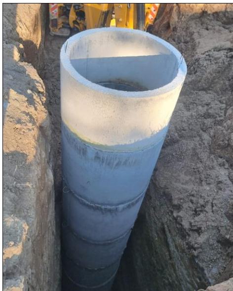
Picture 7: Placing precast concrete elements is a lot a faster and simpler way of securing the well wall (Foto. N.Urošević)
