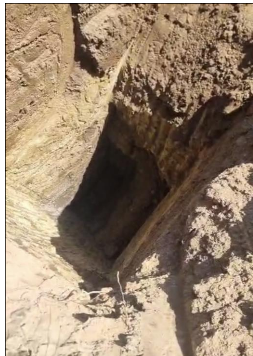
Picture 6: Water at a depth of 8 m, digging done (Foto:N.Urošević)
