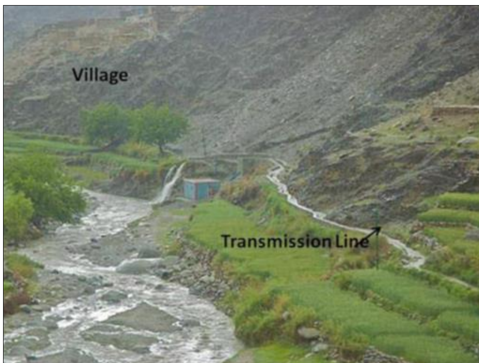
Fig 6: A 7kW micro-hydro project in Padisaw village (Afghanistan) using a run-of-river [38]
