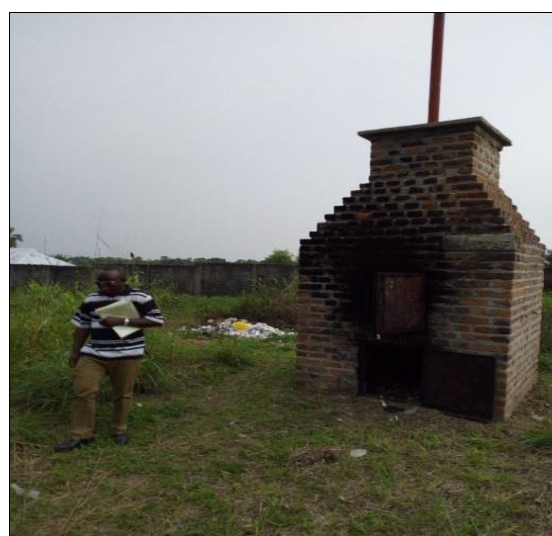
Fig 6: Incinerator down next to an unsecured and open DBM storage facility
