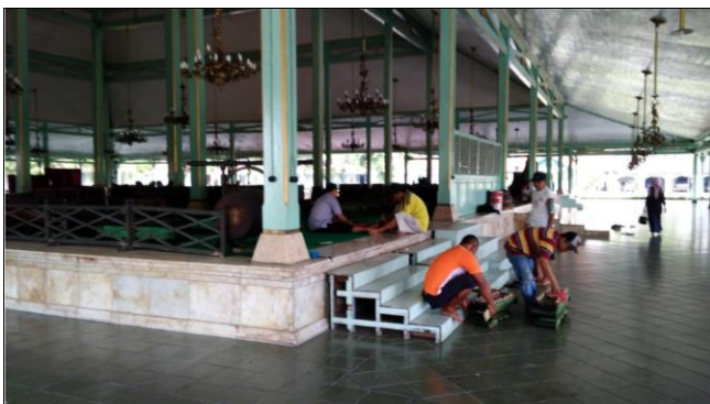
Fig 10: Floor Lined Pendapa and Pedestals-Marble
