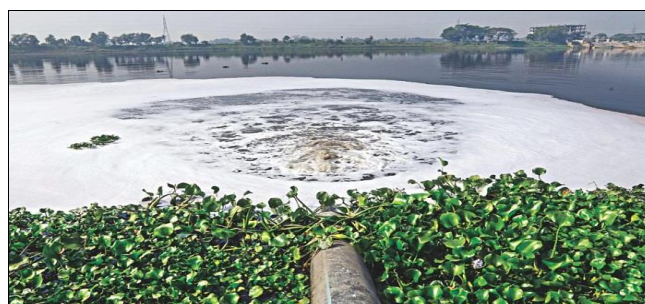
Picture 3: Direct Discharge of Partially treated effluents into the Dhaleswari River (The Daily Star, 2019) [17]
