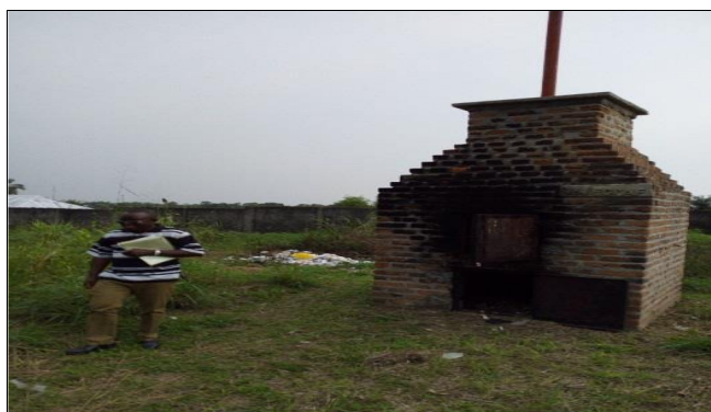
Fig 6: Incinerator down next to an unsecured and open DBM storage facility
