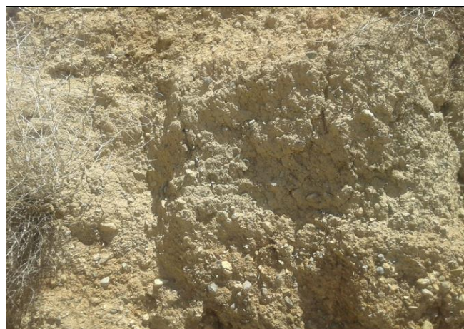
Fig 3: The remains of a wall in the old place of Mubarekeh
