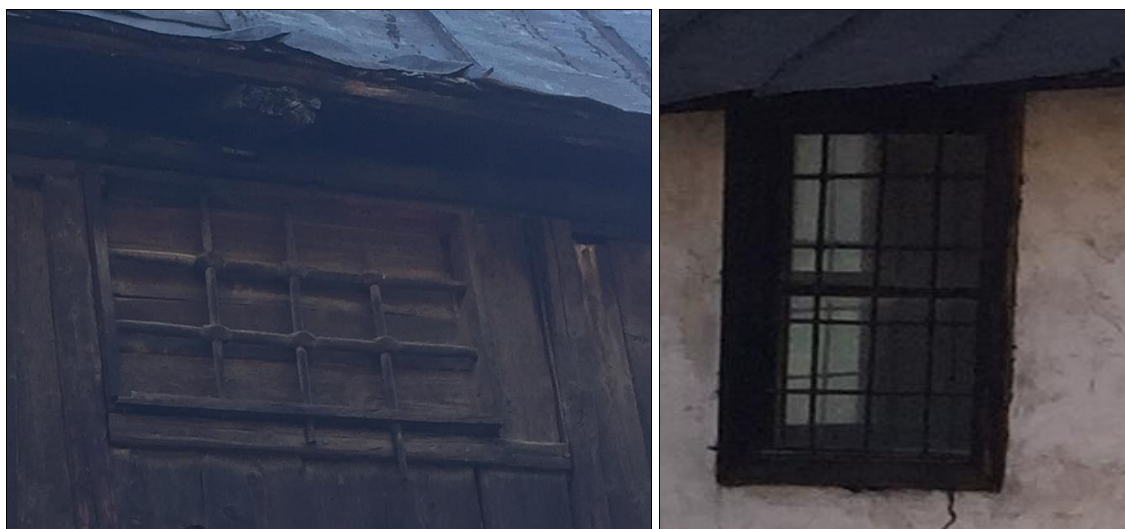
Fig 17: Korkut family house in Travnik. Window on the divanhana with wooden 'demirs' and on the porch with iron 'demirs'
