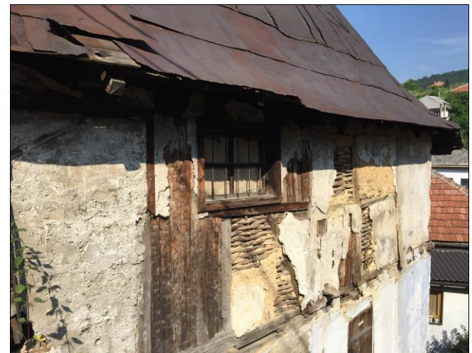
Fig 11: Korkut family house in Travnik. Construction and materialization of floor walls (right)
